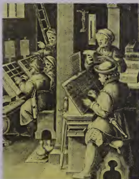
Above, engraving, c. 1600, of a printshop, showing the setting of type by hand.
