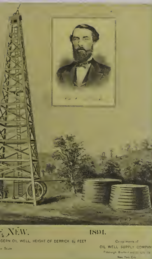
American oil derrick, 82 ft. high, erected in 1891. Insets show the first derrick put up in America (1859, near Titusville, Pa.), 34 ft. in height, and Col. E.L. Drake who drilled the well.
