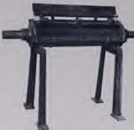
Hancock masticator, used for 'plasticizing' rubber in Britain before 1850.
