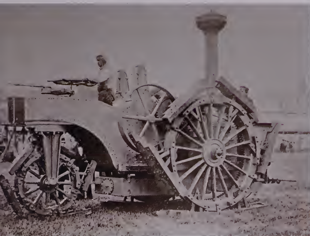
Early attempt at an 'artificial road' – Boydell's steam-tractor of 1854, one of the forebears of the caterpillar track.
