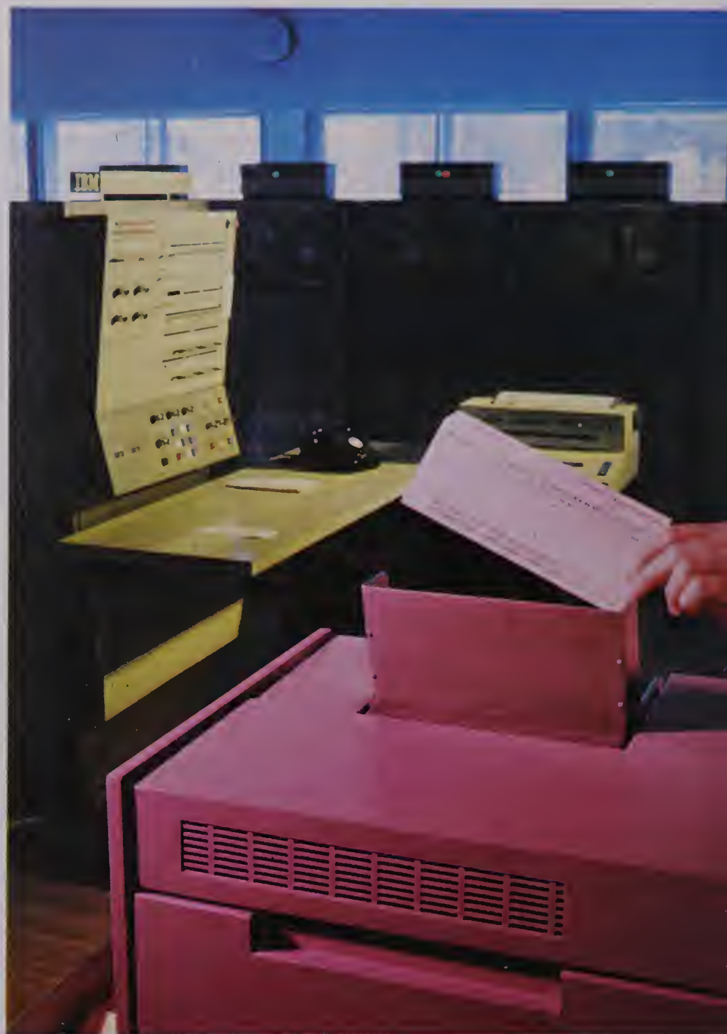
IBM System/360 computer. The data on which the computer, already programmed, is to work are being fed in by means of a punched card. The holes are translated into pulses of electric current.
