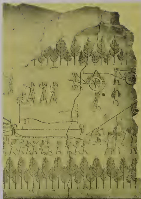
Relief representing the construction of Sennacherib’s palace at Nineveh: a statue of a winged human-headed bull is being levered up a slope.
