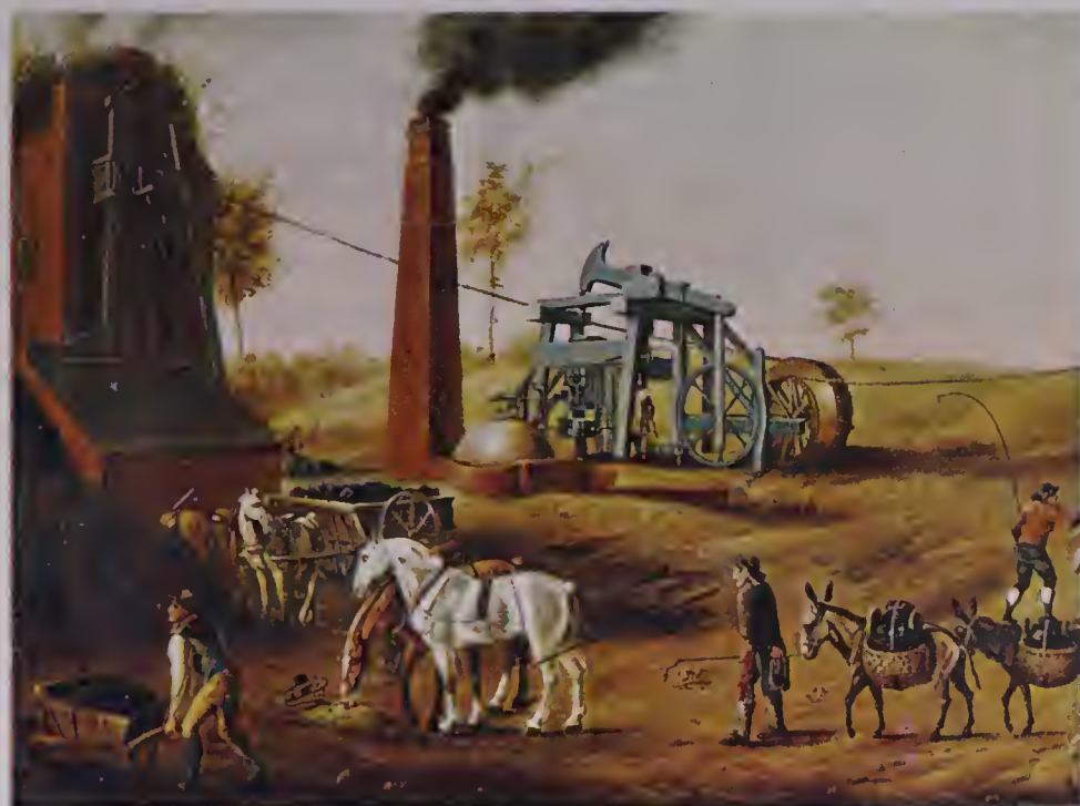
Newcomen's steam engine, which he erected at Coneygre Colliery, Staffordshire, in 1712.
