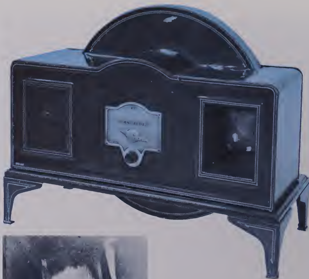
John Logie Baird's 'disc televisor' of the 1930s. In 1937 Baird's mechanical system lost out to the faster and better electronic system.
