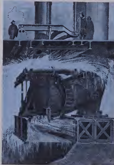
Turbine in the first Niagara power station. A contemporary engraving gives a vivid impression of the force involved.
