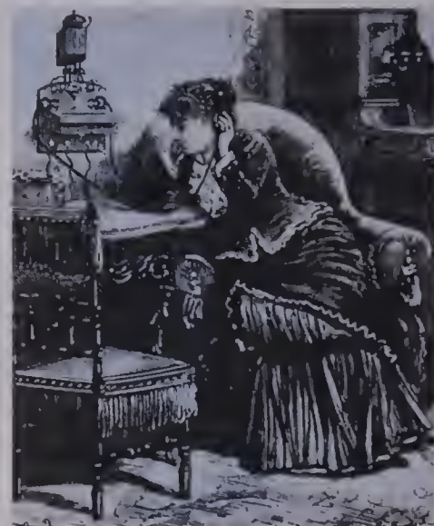
Reception through two earpieces of an opera performance, by Ader's stereophonic system.
