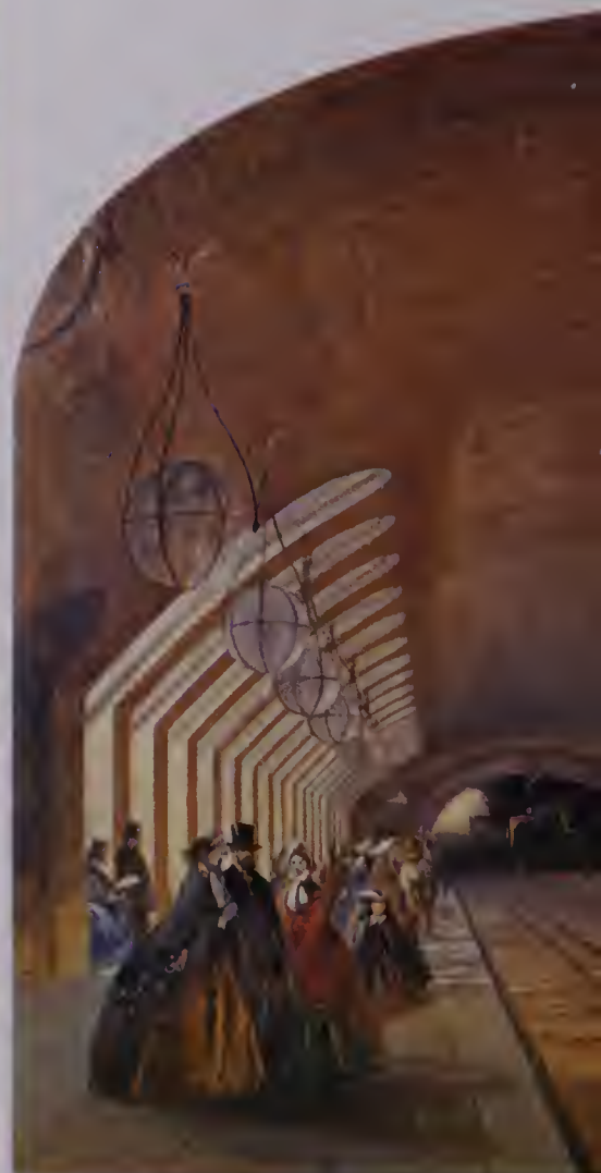
View of the Metropolitan Railway at Baker Street Station, London. Chromolithograph, 1868.
